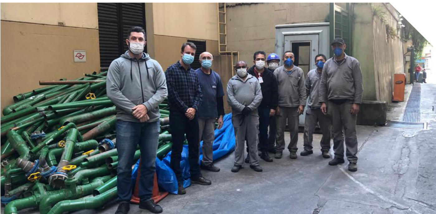
REPLACEMENT OF COPPER PIPING WITH PPR PIPES
